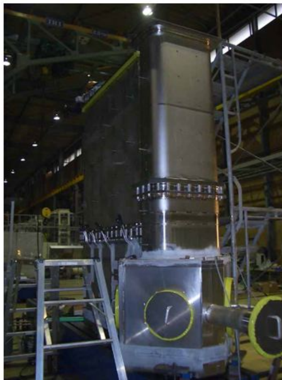
Installation of Alignment Plates XY \pm 0.1\text{mm} Precision Level \pm 0.1\text{ mm}
